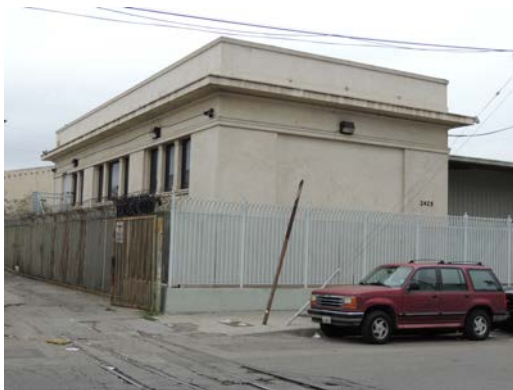
Address: 2417 E Porter Street Name: Edison Electrical Substation Date: 1911
