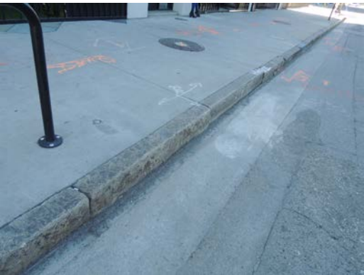
Name: Downtown Los Angeles Industrial Historic District Description: Granite curb
